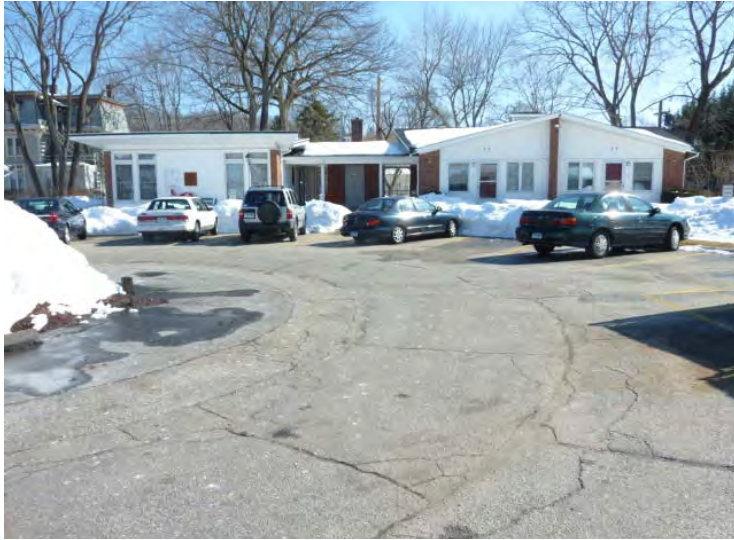
Asphalt drive at the Community Center and site-wide is in poor condition.
