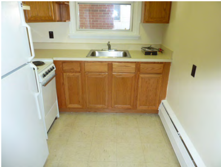
GFCI outlet is required at counter to right of sink and is shown to be installed in Year 1 where missing.
