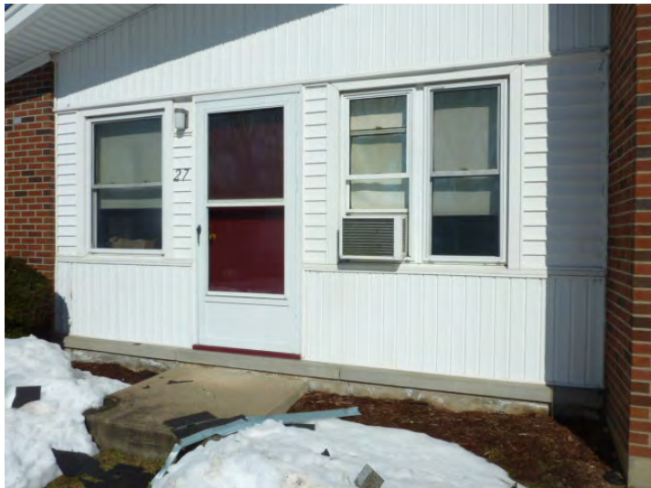
Typical front elevation with storm doors, entry doors, windows and vinyl siding typically in good condition and shown to be replaced mid-plan.
