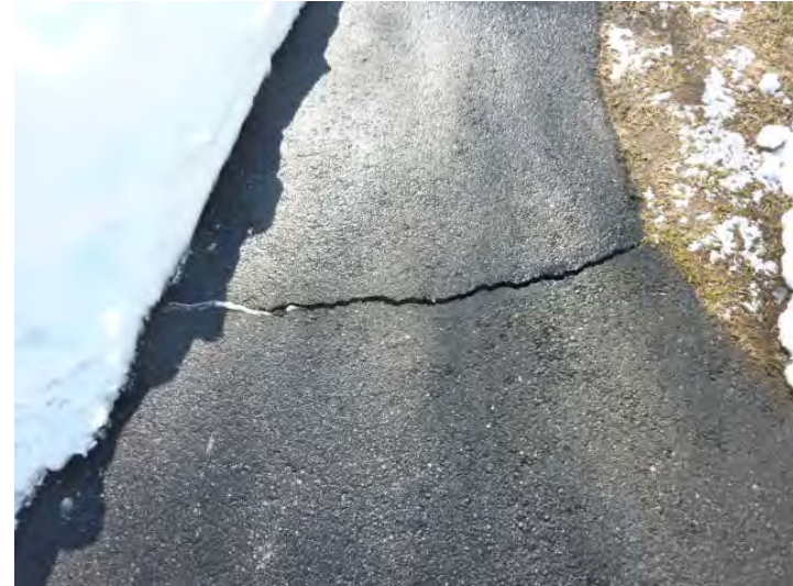
Typical cracking at asphalt walks.
