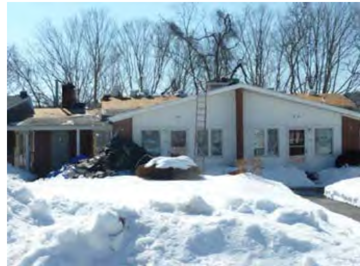
Reroofing with new asphalt shingles was ongoing on the day of our visit.
