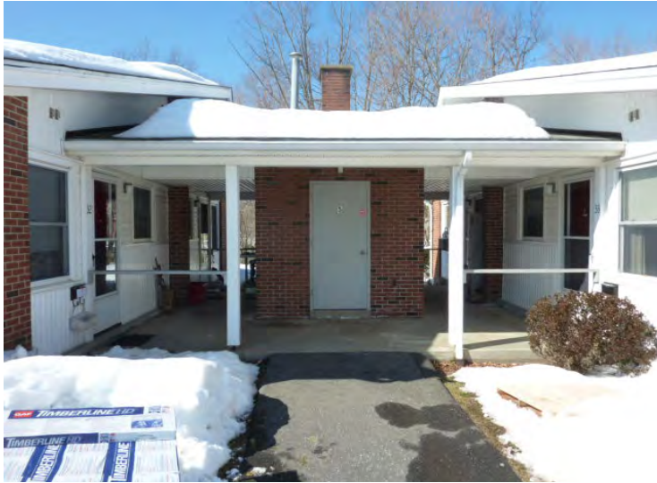
Mechanical Room with the building boiler and DHW heater is located between each pair of 4 unit buildings on a concrete patio.
