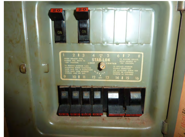
Stab-Lok electric panels are shown to be replaced in Year 1.
