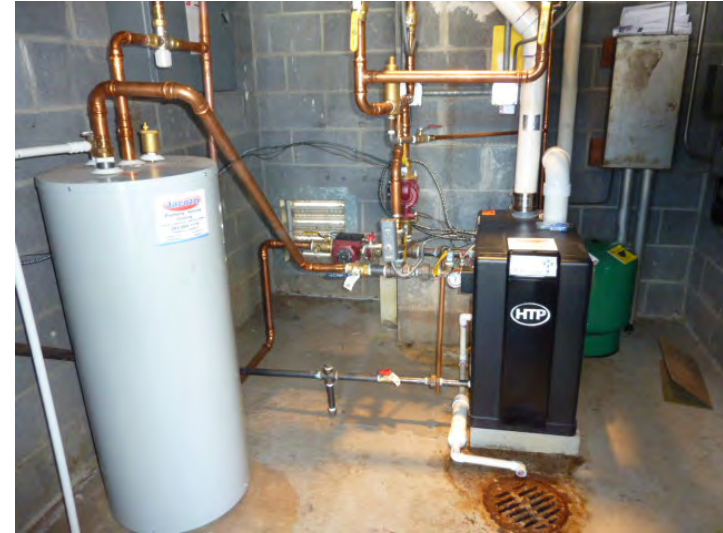
Installation of new gas-fired instantaneous indirect boilers and DHW heaters is ongoing and is shown to continue over the plan.
